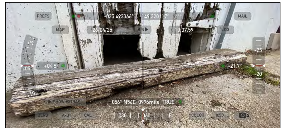
Looking at the east facing door with significant gaps for ember ingress on the existing building.
