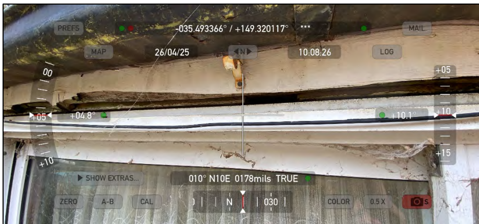
Showing gap above the window into the interior of the building
